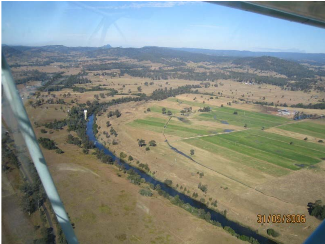
Photo: Coles Crossing on the Mary River – (Goomong pumping station on bend of the river) - part of proposed water supply for NPI stage 2
